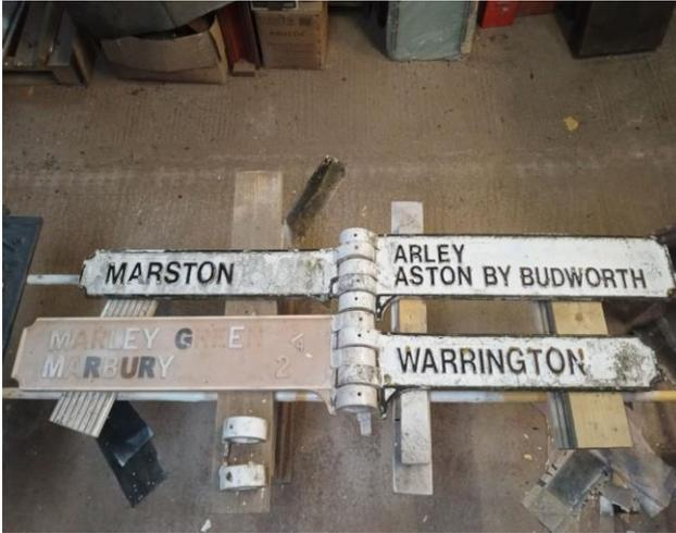
This pattern can be seen in the picture (left) before having its new letters applied, being laid out in its collar sequence to ensure everything would fit together as it should.
